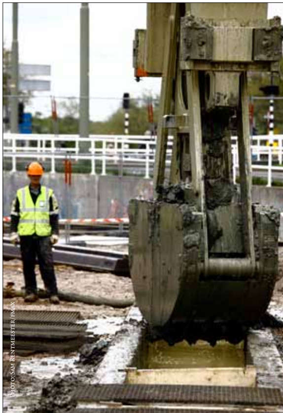
Construction builders dig trenches for the diaphragm walls.
